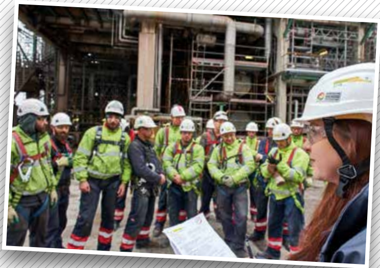
BUCHEN and XERVON had a team of over 1,000 operatives working on site at the plant during the TAR 2018
