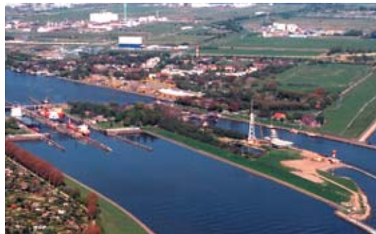
SAVA is located on an area covering seven hectares in the industrial area of Brunsbüttel, near to the Elbe port and the Kiel Canal.
